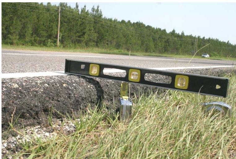
*Fig. 3 Shoulder “dropoff” is 5 inches. Many drivers would have trouble if they left the pavement in this area.*
