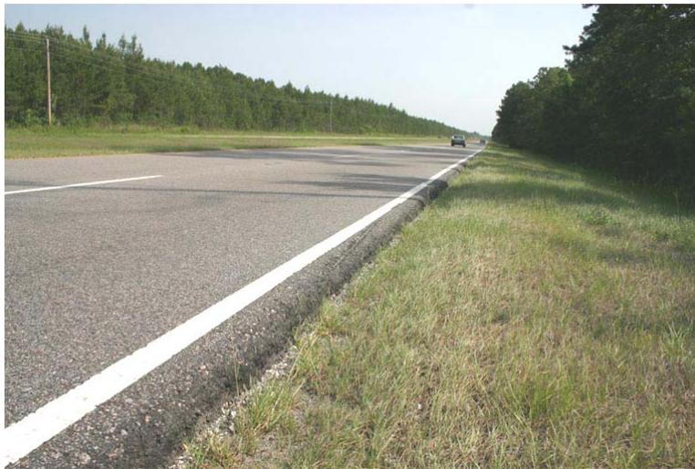
*Fig 2 Shoulder dropoff on U.S. Highway 17 near Georgetown, South Carolina. Note the scrape at the pavement edge.*
